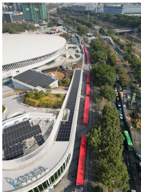
Figure 3. Shenzhen Longhua Culture and Sports Center with photovoltaic panels installed
