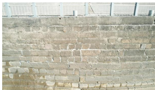
Figure 3. Close-up view of the glutinous rice mortar repair
