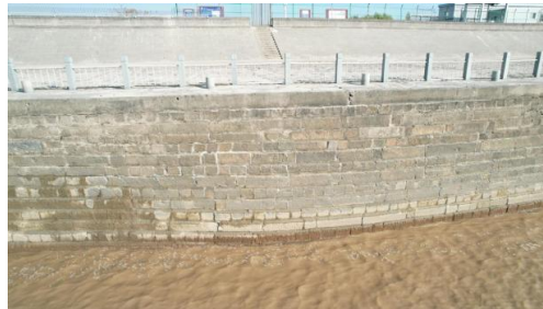
Figure 2. Overview of the glutinous rice mortar repair
